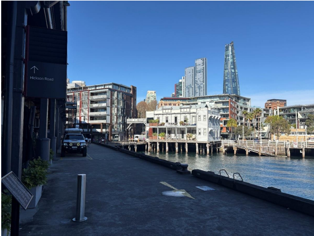
Figure 4: View south along the west elevation of Pier 9
