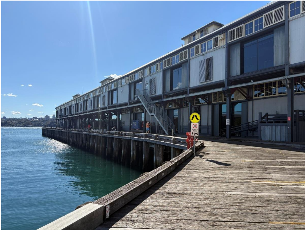
Figure 2: Western elevation of Pier 9 when viewed from the south. The building's external weatherboard cladding as well as pier and beam structure are visible.
