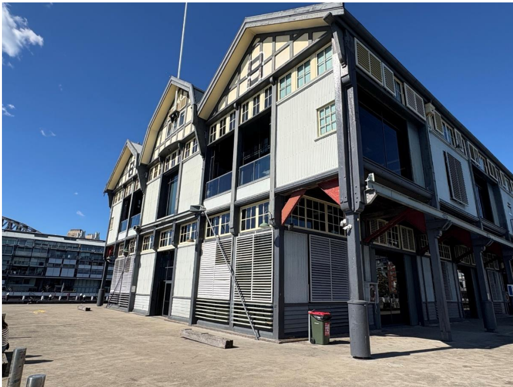
Figure 5: Northern elevation of Pier 8/9
